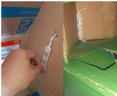
Gambar 5. 17 Instalasi lampu led strip
